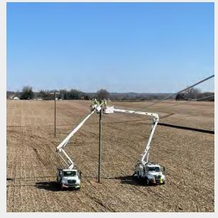
Pictured: Lineworkers installing overhead line to new headquarters site. Photo courtesy of Andrew Ruder.
