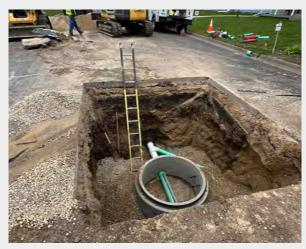
Pictured: A sewer manhole being replaced on West Street after it had started to collapse. It was originally installed over 60 years ago.
